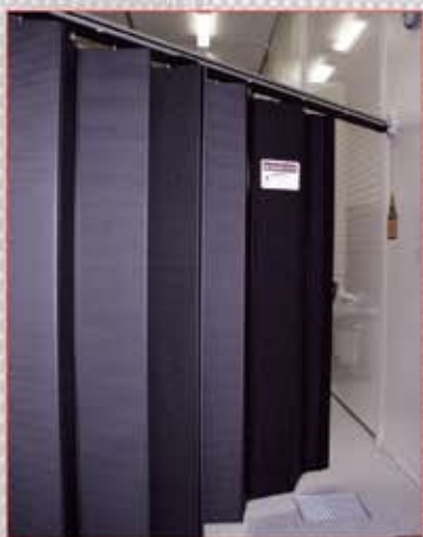
short curtain segment to shield entry
